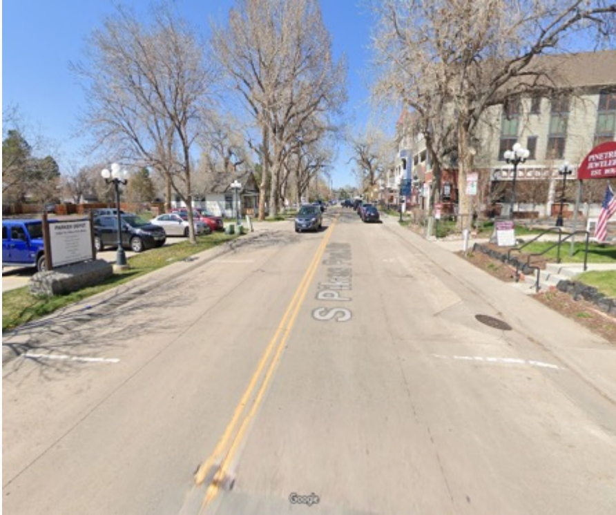
Existing Conditions Looking North
