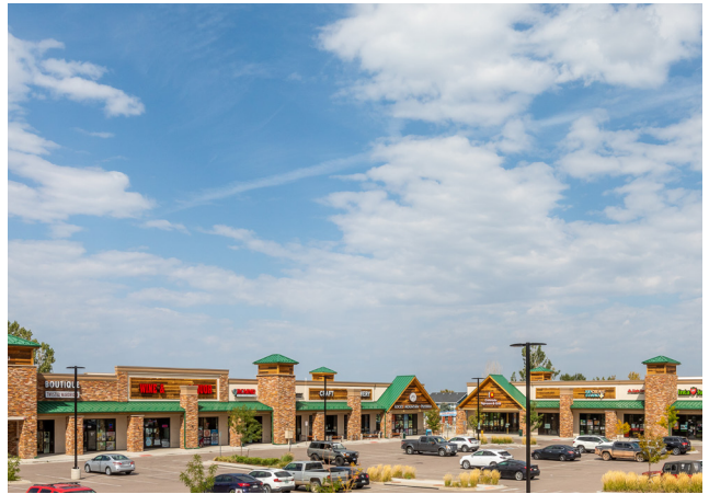
Shopping center in Parker. Photo from the Town of Parker.
