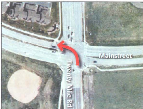
The red arrow turning movement at Mainstreet and Twenty Mile Road has insufficient capacity.
